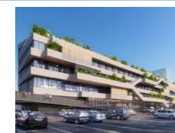
Construction of prefectural facilities
