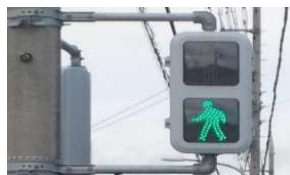
Switching to LED traffic lights
